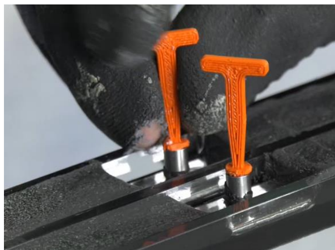
Fig. 11 SWS Air installation into insulating glass unit
