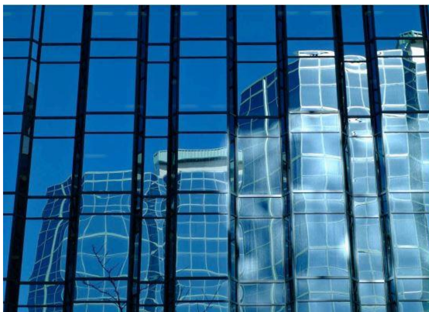
Fig. 26 Distortion effect, depending on concavity/convexity of glass panes due to overall bow and roller wave of toughened glasses, etc.
